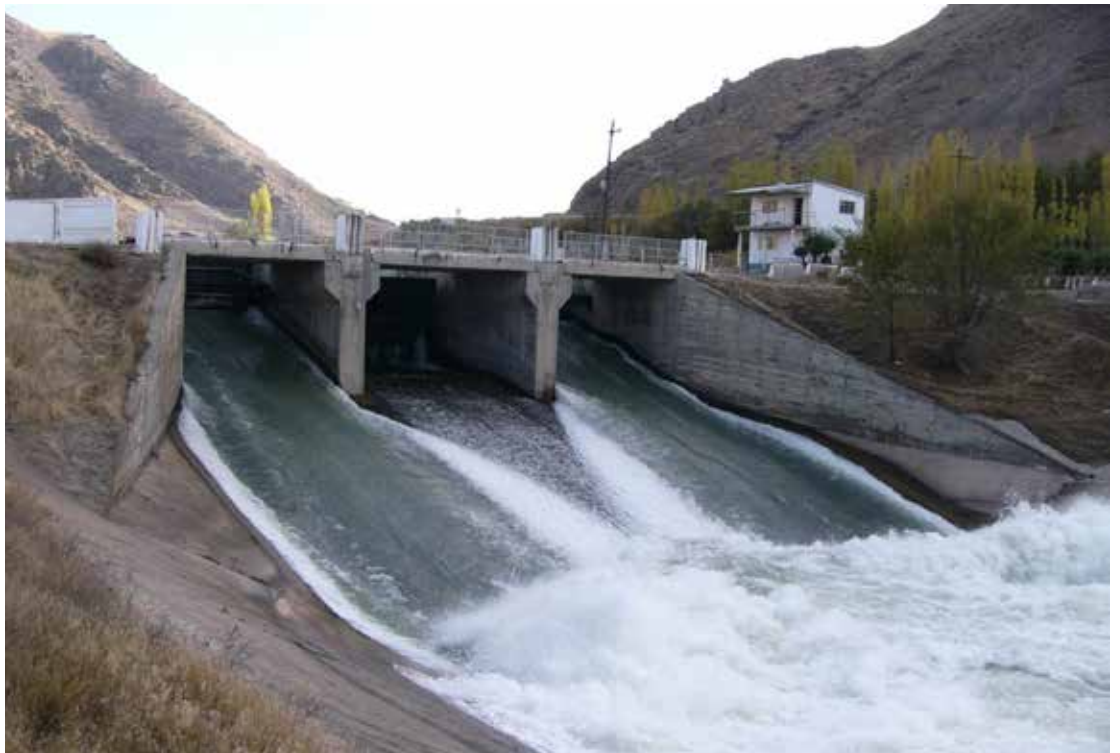
Promotion of Transboundary Water Cooperation between Kyrgyzstan and Kazakhstan: Hydraulic distribution structure below the Kirov reservoir. © SDC
