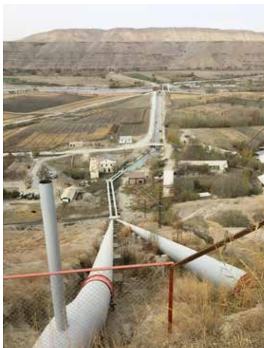
Water pipelines, Aksu Watershed, Tajikistan, ©SDC
